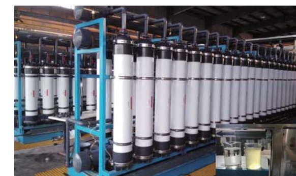
SMBR for industrial wastewater
