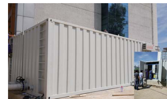
SMBR container for industrial wastewater
